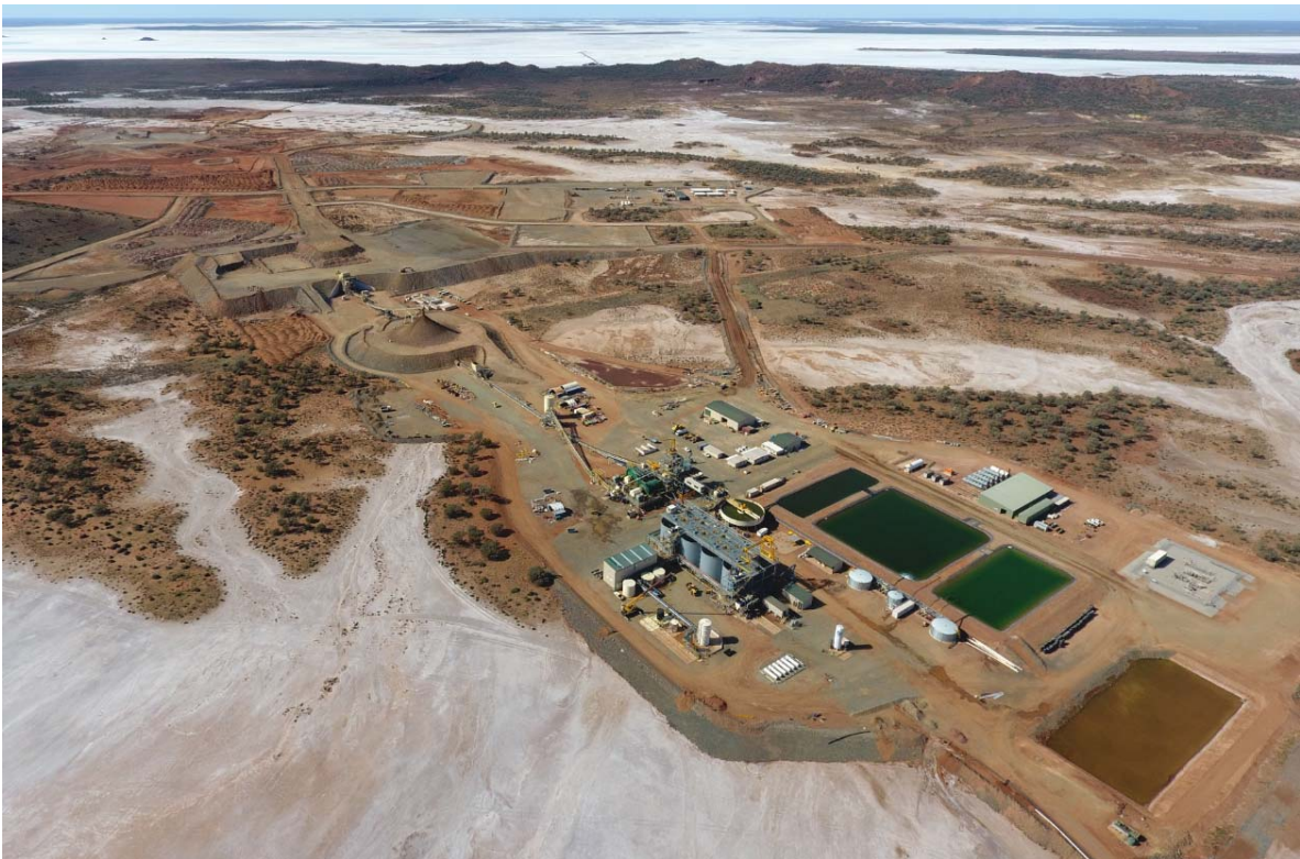
Figure 3: Corresponding photograph to Figure 2, showing the completed 2.5Mtpa treatment plant. This photograph was taken exactly 10 months after the photo shown in Figure 2, on the 24 th March 2018.
